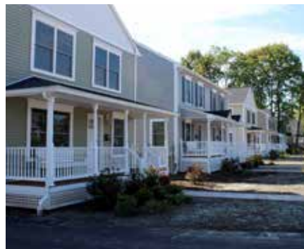
Completed six units on Main Street-Hartford
